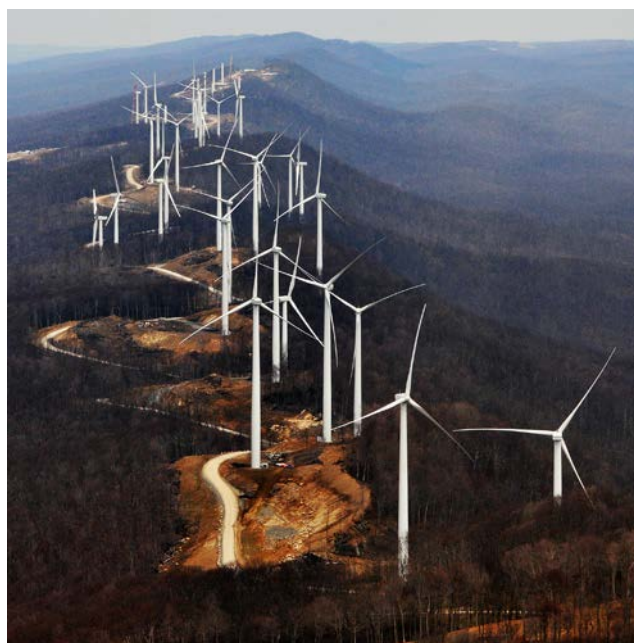
Wind turbines on Laurel Mountain
